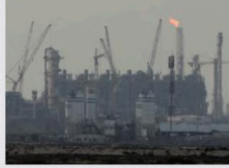
MISSILE ATTACK. QatarEnergy's LNG plant was damaged last month REUTERS
