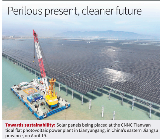
Towards sustainability: Solar panels being placed at the CNNC Tianwan tidal flat photovoltaic power plant in Lianyungang, in China's eastern Jiangsu province, on April 19.
