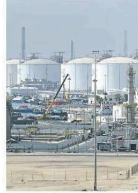
LNG facilities in Ras Laffan Industrial City in Ras Laffan, Qatar.
