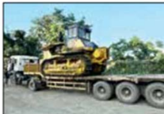
Mobilisation of heavy equipment for capping of well
