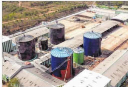
Compressed biogas plant. File photo
