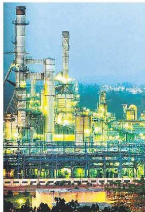
Reliance has an ethane cracker in Dahej, Gujarat, to produce ethylene. BLOOMBERG
