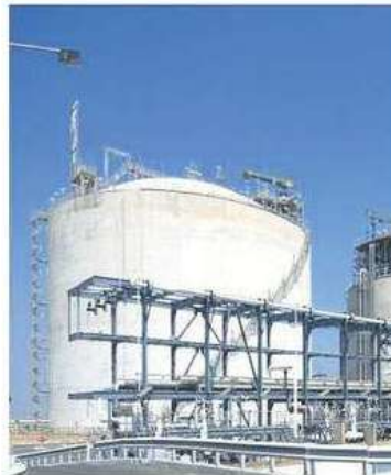
India plans to renew efforts for interconnectivity of the gas grids of the three nations.
